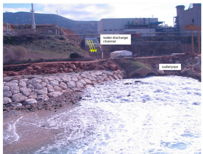
Figure 7 Discharge channel and outfall water, Deir Ammar (Beddawi power plant)
