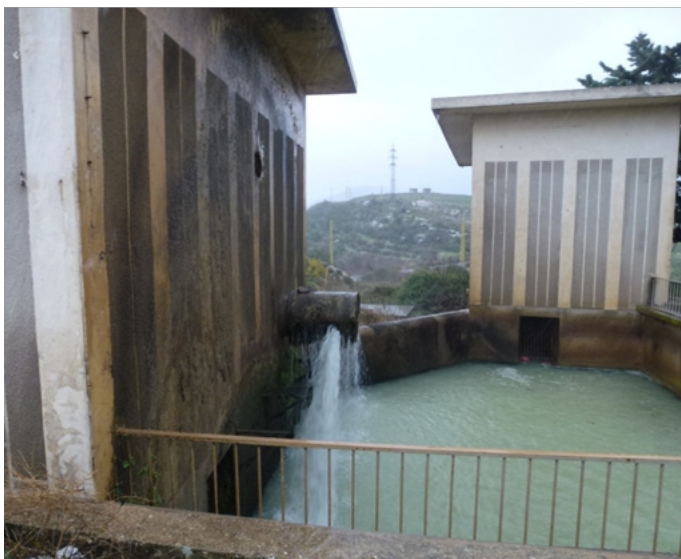
Figure 15 Falouss irrigation site– Discharge pipe at BC2 location
