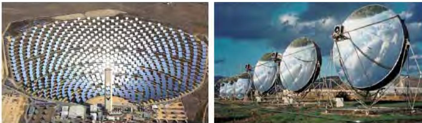
Figure 10. Point-focusing systems: Left: Solar Tower plant PS10, 11 MWe in Seville, Spain; 624 so-called heliostats, 120 m<sup>2</sup> each, focus the sunlight onto a receiver on top of a 100 m high tower (Abengoa, 2010). Right: Dish Stirling prototype plants of 10 kWe each in Almería, Spain; diameter 8.5m (PSA, 2010)
