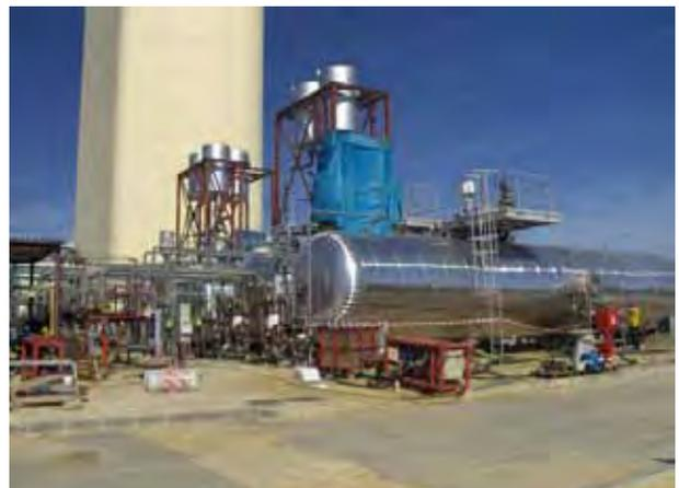
The four Thermal storage tanks for PS10
