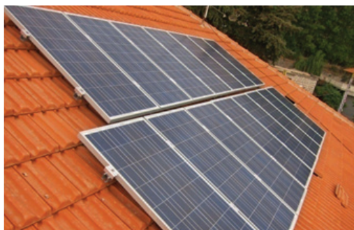
Figure 22. PV modules fastened to the tilted roof structure. Installation done within the CEDRO project (Source: CEDRO project site)
