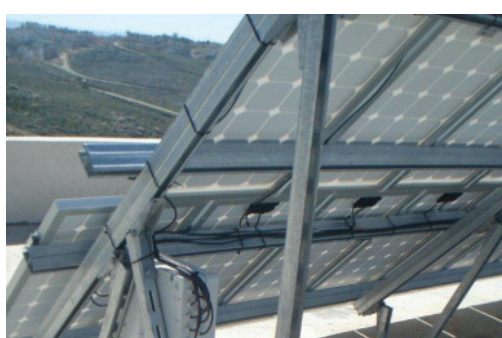
Figure 24. Anchored structure. Installation in Kfor done within the CEDRO project (Source: CEDRO project site)
