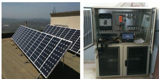
Figure 36. Back up grid tied PV plant with storage. The cabinet for storage and power conversion is easily accessible, well ventilated and the PV generator roof mounted in two rows. Kfarshouba Intermediate public school, South (Lebanon) – Pilot project implemented by the CEDRO project
