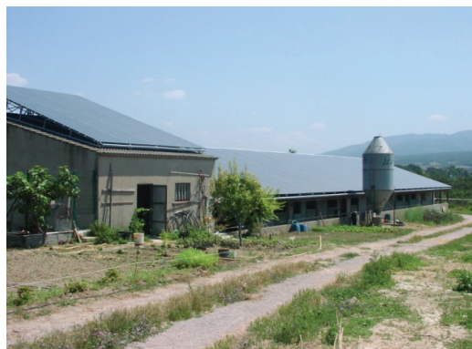
Figure 26. Grid-connected PV generator integrated on roof according to the space available and characteristics of the location (Source: TTA)
