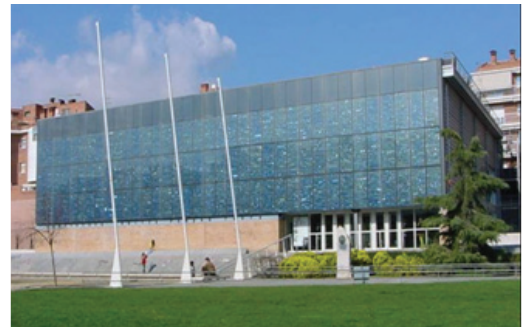
Figure 19. PV installation functionally integrated into the building façade. Library in Mataró, Spain (Source: TTA)
