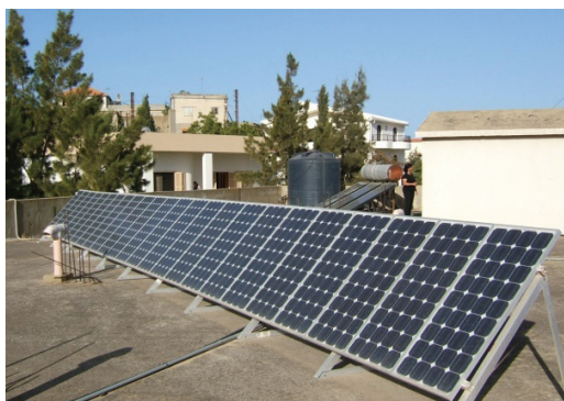
Figure 29. PV installation on the roof of El Tleile public school developed within the CEDRO project. The PV modules face 20° east and 45° tilt (Source: CEDRO site)
