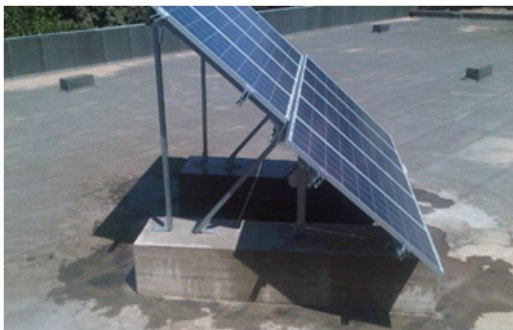
Figure 21. Ballasted structure with concrete blocks on flat roof. Installation in the army barracks site done within the CEDRO project (Source: CEDRO project site)
