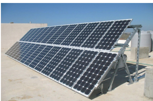
Figure 23. Structure anchored to the roof. Installation done within the CEDRO project (Source: CEDRO project site)
