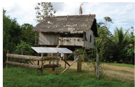
Figure 5. Autonomous AC PV micro plant (400Wp) in a rural community in Ecuador (Source: TTA)
